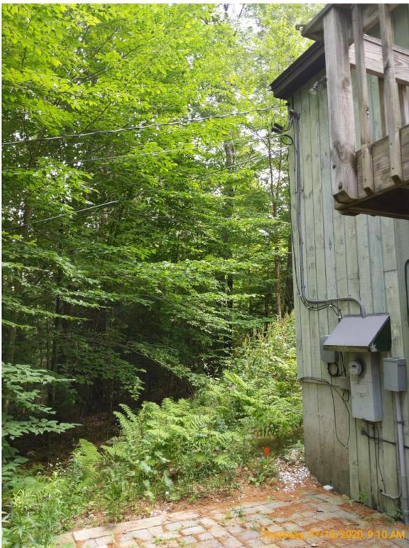
**181:** The overhead service-drop conductors had inadequate clearance from tree branches. This condition should be corrected by a qualified contractor or the utility service provider to avoid abrasion and damage to the conductors. Work around the service conductors should be performed by a qualified personnel only. Injury or death may result from attempts at correction by those without proper qualifications. There are tree branches resting on the service line
