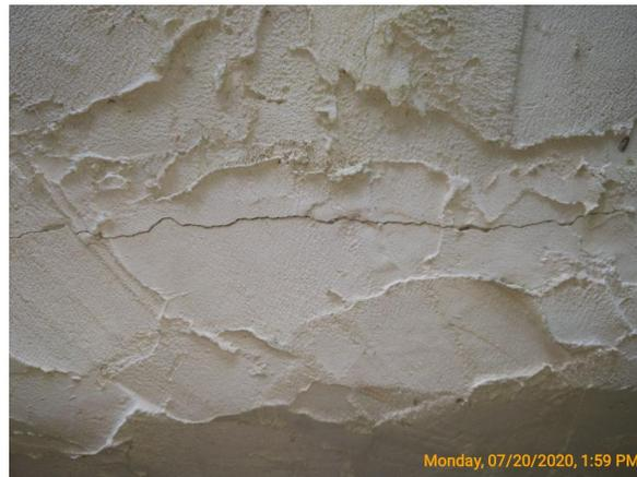
**52:** The wood frame chimney structure was covered with stucco. This was used to enclose the chimney pipes for the wood burning insert.
